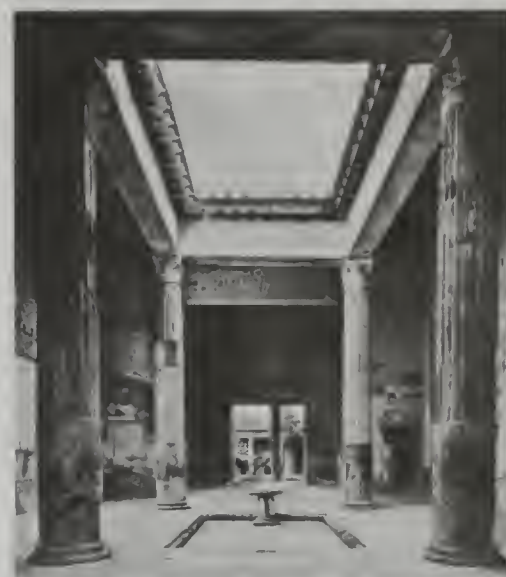
Atrium with impluvium and compluvium of the "House of the Silver Wedding," Pompeii, Italy, c. 1st century AD
